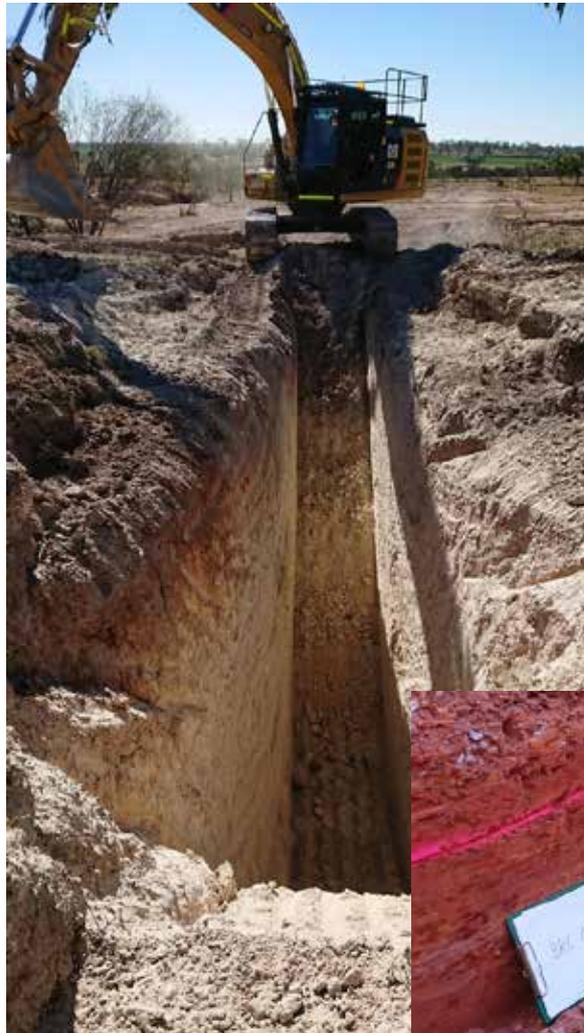
**Figure 27:** Photographs showing the free digging nature of the oxide material in the top 4 to 5 metres and also the target unconformity. Samples were taken approximately 1.5 metres above to 0.5 metres below the unconformity. There are large volumes of free-digging material across the Blackridge project.
